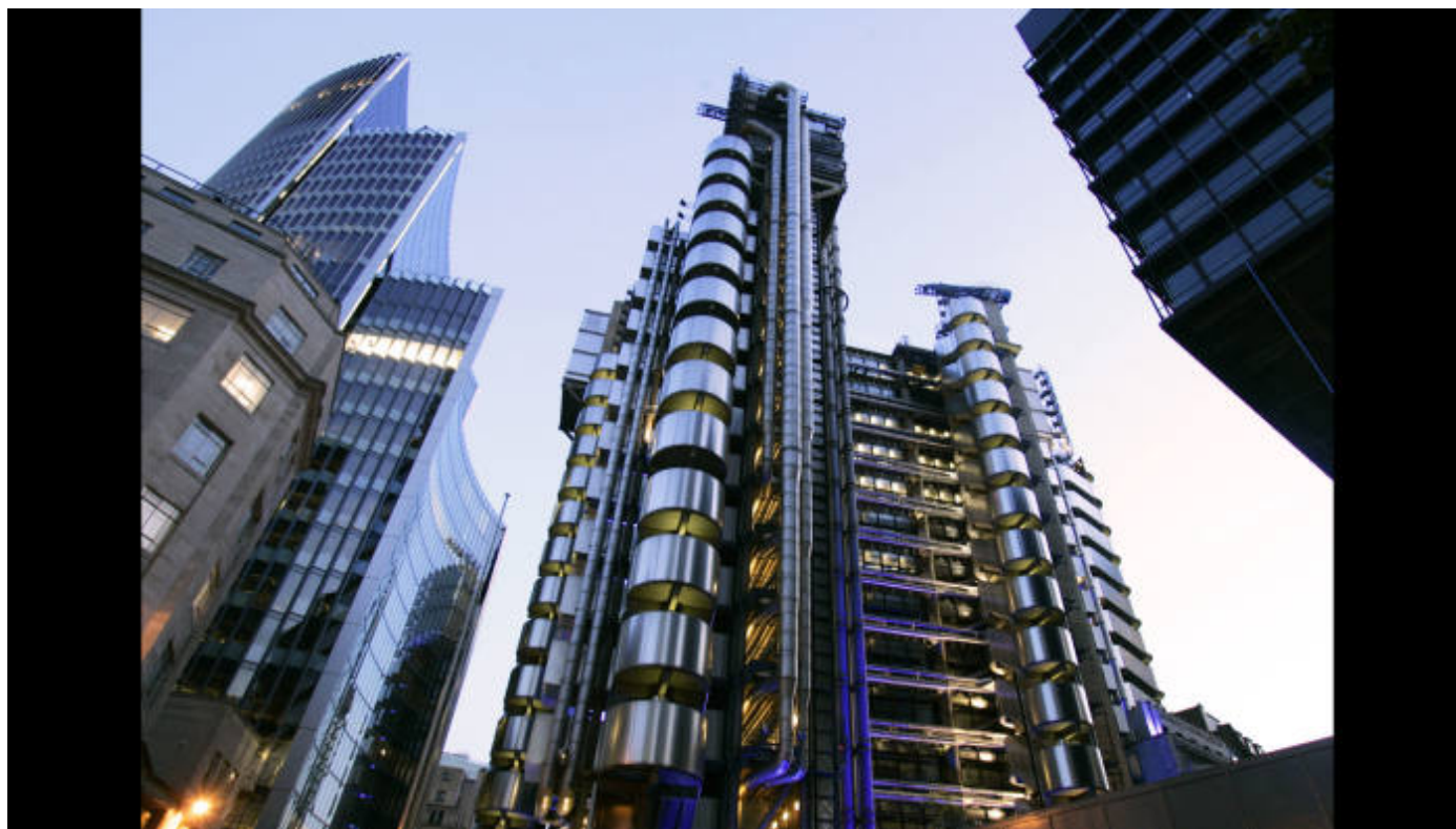
Example: Llyods's Building, London. Architect: Richard Rogers
