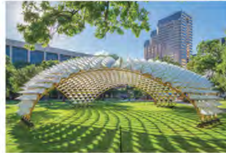
FIGURE 1: 'GRID SHELL IN THE PARK', SAN ANTONIO, USA
