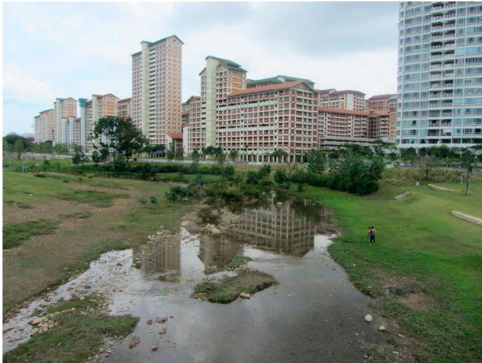
Figure 12. Concrete from an old canal is recycled into the new Kallang River, Singapore. Source: Peter Newman.
