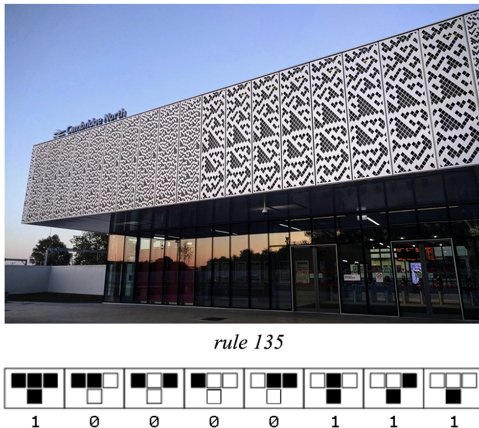
Fig. 9 Application of Stephen Wolfram's rule 135 in the design of Cambridge Railway station, Cambridge, UK. Top: façade of the station. Bottom: rule 135 that were used to generate the façade pattern.
